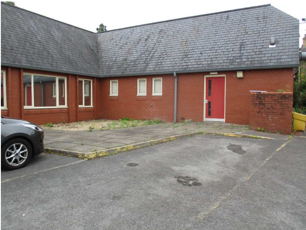
Photo 2 – Pedestrian access route
